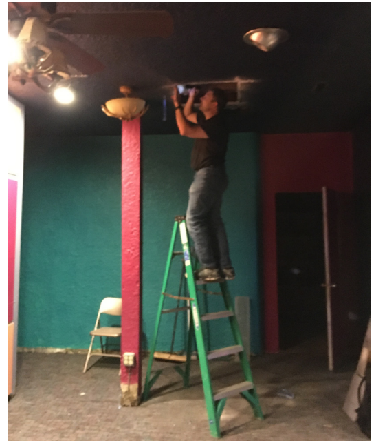
LOBBY FINISHES AND LIGHTING
