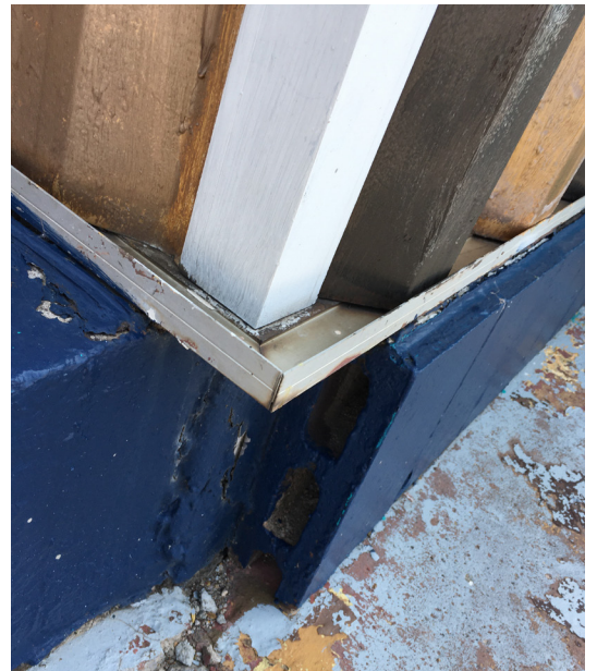
NON-HISTORIC TERRACOTTA BASE ON SIDEWALK
