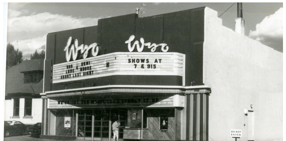
1986 FACADE PHOTO, COURTESY OF THE LARAMIE PLAINS MUSEUM
