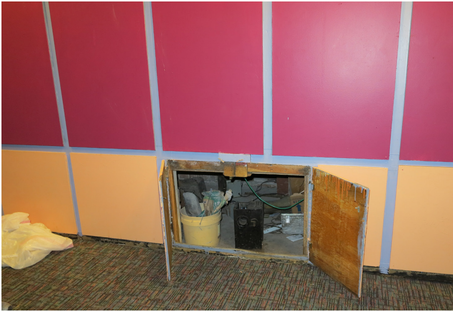
LOBBY: NON-HISTORIC WALL FINISHES ADDED IN 2014
