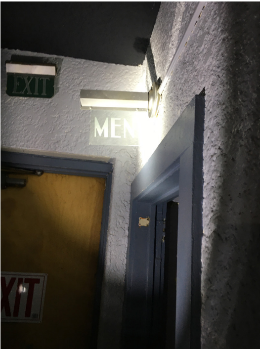
EXISTING HISTORIC LIGHT TO REPAIRED & REINSTALLED
