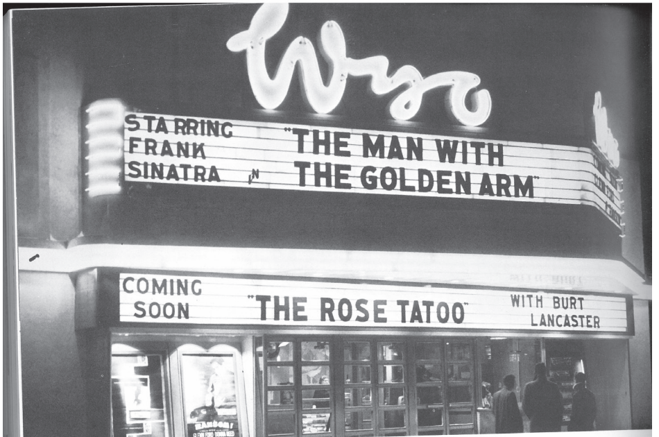
1955 FACADE PHOTO, COURTESY OF THE AMERICAN HERITAGE CENTER
