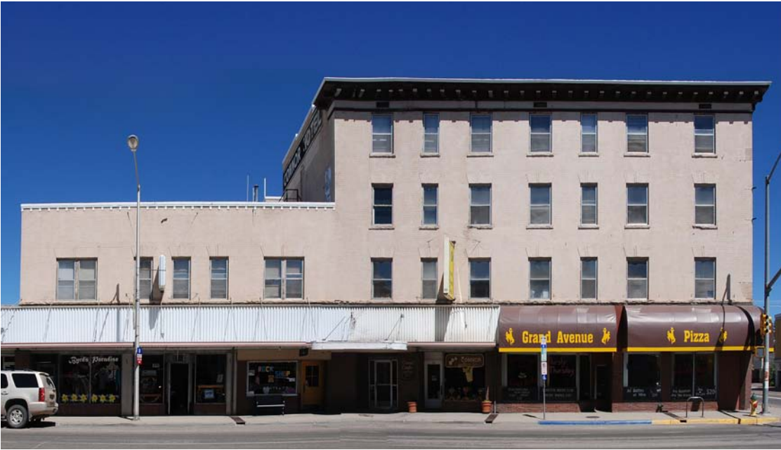
Fig. 3.4: Existing photograph of Connor Hotel.
