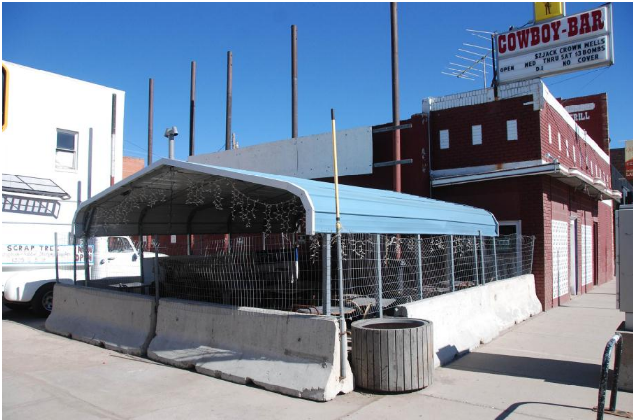
Fig. 3.7: Photograph illustrating the Cowboy Bar's unattractive outdoor dining area at the highly visible intersection of Grand Avenue and 3rd Street.
