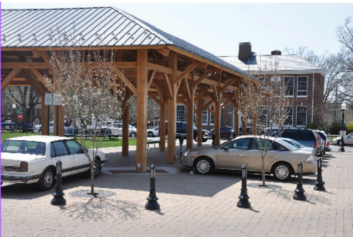
Fig. 3.36: Precedent photograph showing potential market shed structure. This example is from Blacksburg, Virginia.
