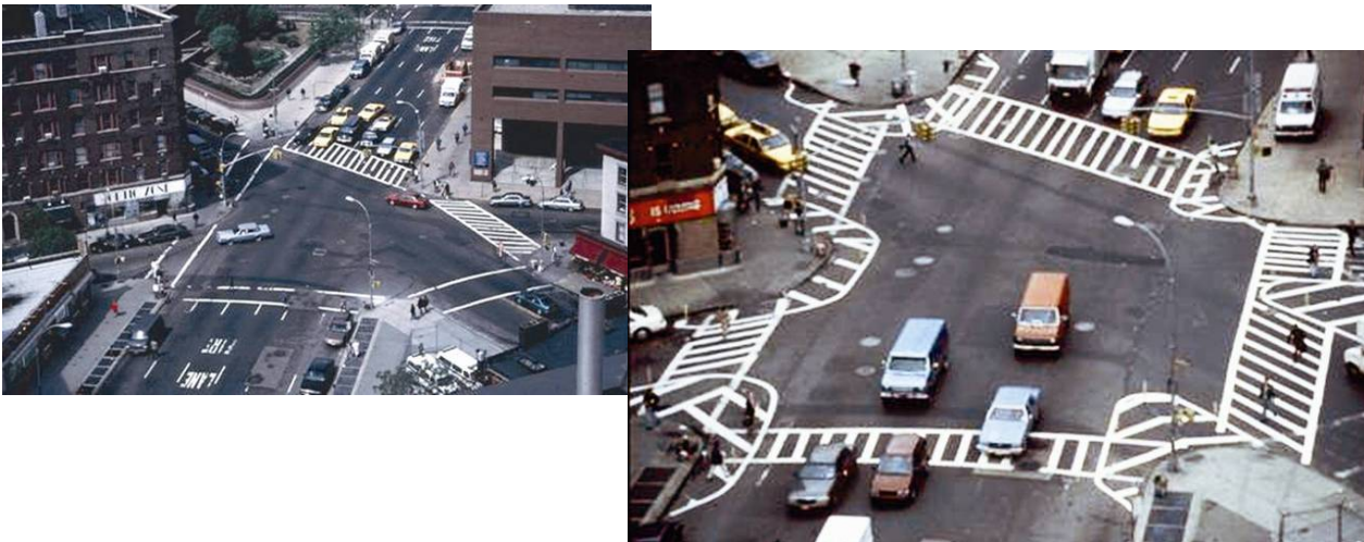
Fig. 2.8 : Before (left) and after (right) photographs illustrating how marking tape can be used to show new road and sidewalk configurations prior to making significant investment in permanent changes.
